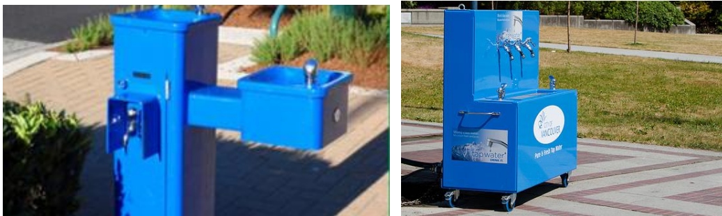
Figure 4 - Example of drinking water fountain (left) and temporary fountain (right) by city of Vancouver
