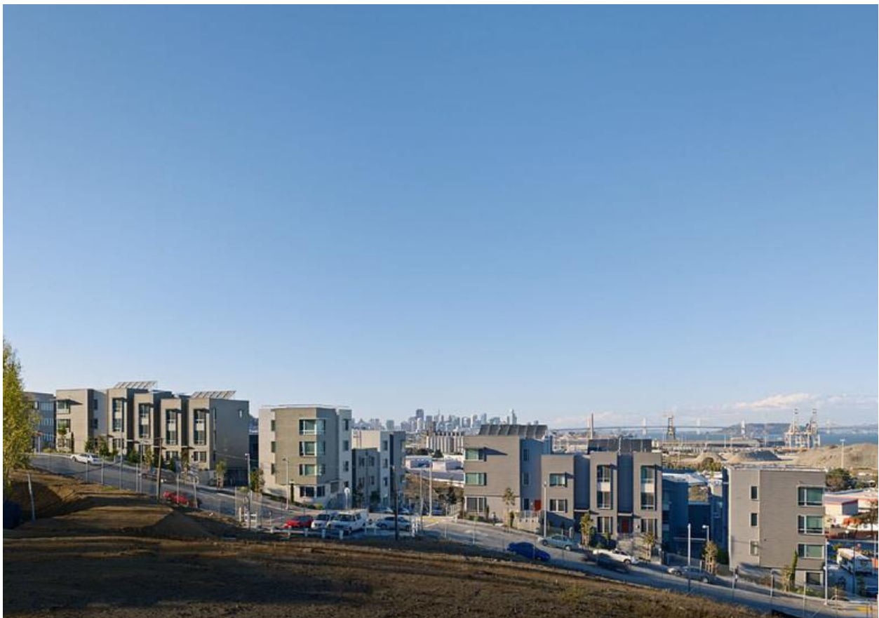
Figure 6. Hunter's View redevelopment, profile shot of the area's steep grades and hills.
