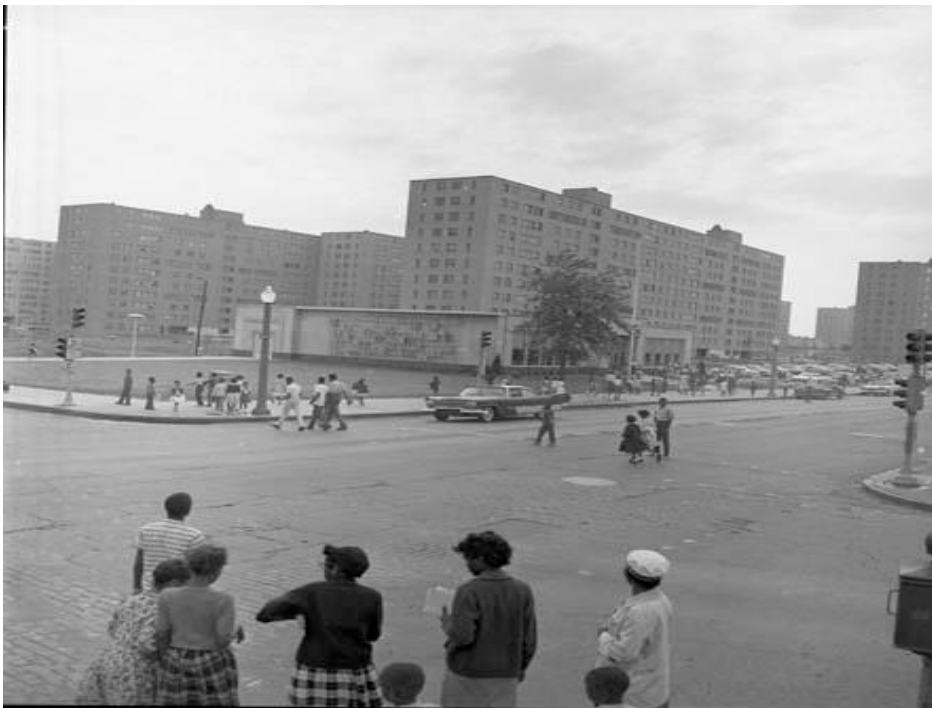
Figure 1. Families and children cross in front of the Pruitt-Igoe homes, four years after their construction.
