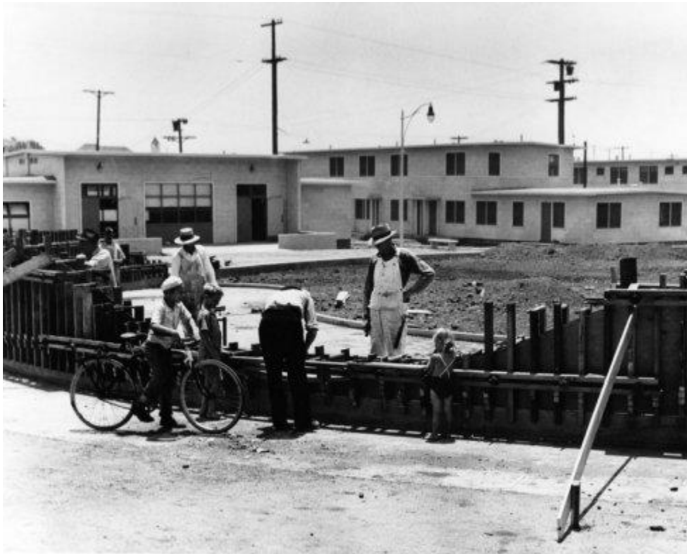
Figure 5. Photograph of Estrada Courts' construction process in the early 1940s.
