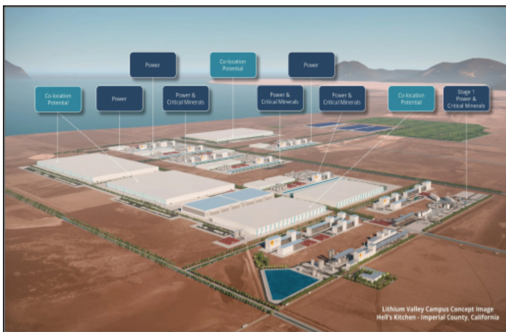
Figure 16. Conceptual illustration of the Hell's Kitchen lithium project in Imperial County, California, showing the proposed full campus layout with co-located auxiliary industrial sites (Controlled Thermal Resources).
