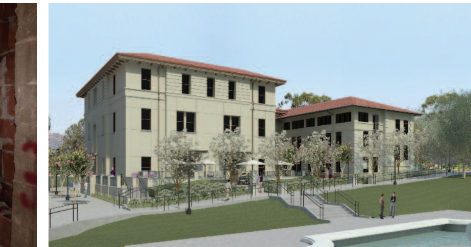
Three phases of Swan Hall: pre-construction, 2009; under construction, June 2011; and an architect’s rendering of the renovated and expanded structure.
