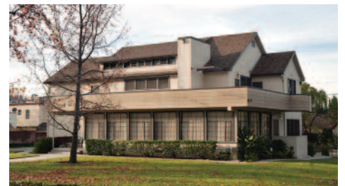
Construction of a new, two-story home for alumni relations is planned at 1599 Campus Road, the former Fiji House and Women's Center (shown as it is today).
