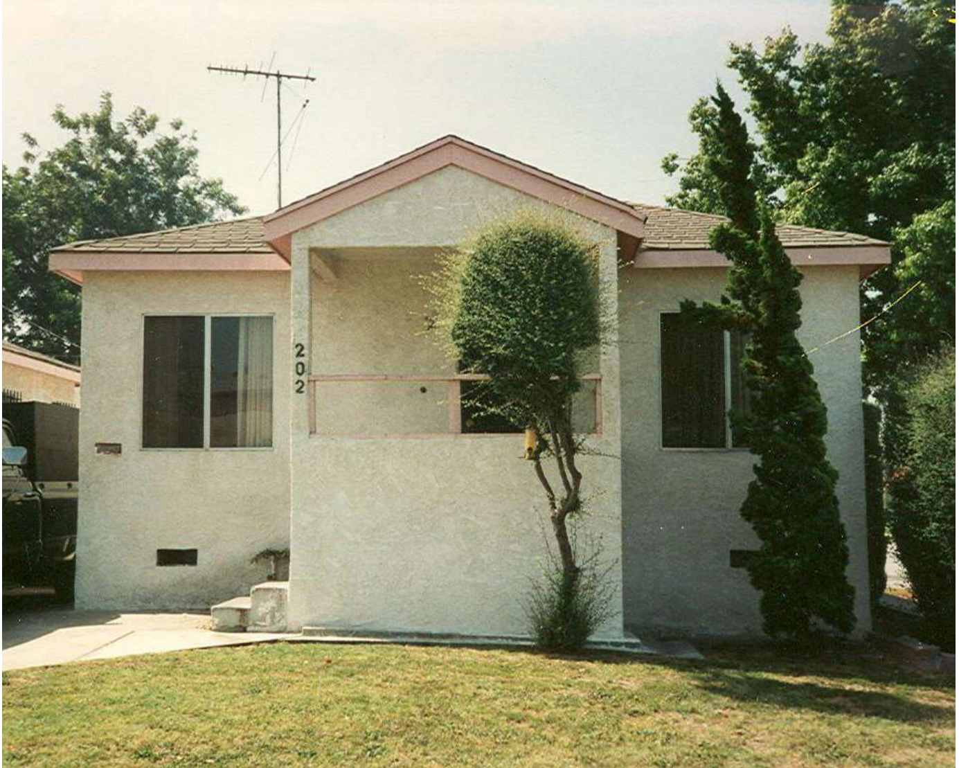
Home in South Central Los Angeles.
